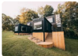
lovePROPERTY homes made out of shipping containers ...
