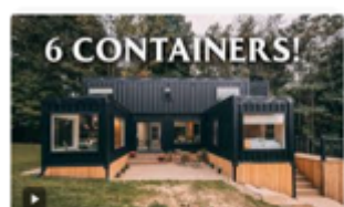
YouTube Massive 6 unit Shipping Container Home ...
