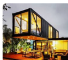
Econtainers 100 Container Houses that will Ins...
